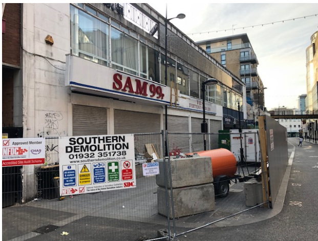
2. Demolition has started on the 5-9 Surrey Street site
