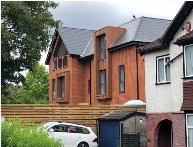
6. An attractive 'contemporary reinterpretation' scheme replacing a single house with a small block of flats on Woodcote Grove Road
