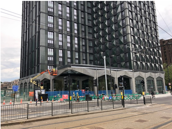
4. Works are nearing completion on 101 George Street
