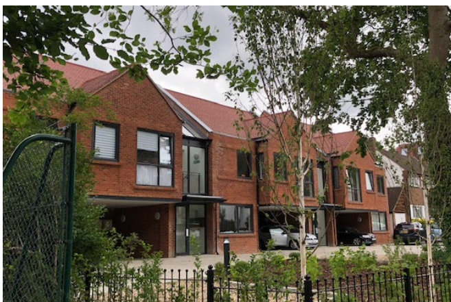
10. The scale of these new homes along Old Lodge Lane is reduced by glazed links between the brick blocks
