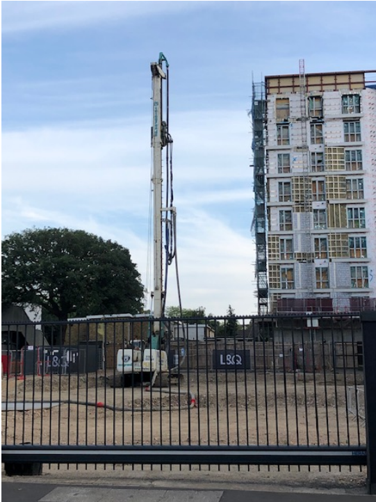
3. L&Q have commenced piling on their site on Addiscombe Road
